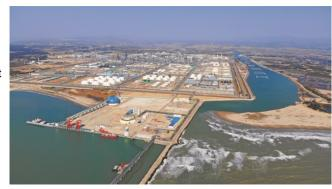
the largest one-time investment project of PetroChina. With an aromatics plant of the largest capacity worldwide and an ethylene plant of the largest scale domestically, the project can process 20 million tons of crude oil, and produce 1.2 million tons of ethylene products and 2.6 million tons of aromatic hydrocarbons annually. Meanwhile, it is built with a 300,000-ton crude oil terminal and a 5000-100,000 ton oil products terminal.
