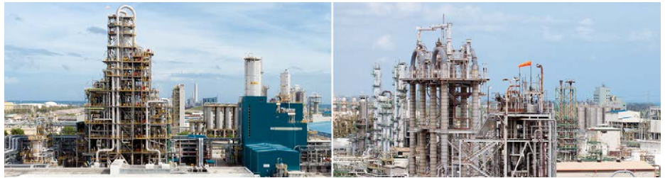
Left: PP Spherizone Plant Right: PP Spheripol Plant 1 - Map Ta Phut, Rayong
