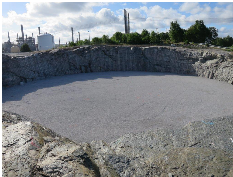
Ground preparations for a new purpose-built, fully refrigerated ethane tank at Borealis site in Stenungsund have started. © Borealis
