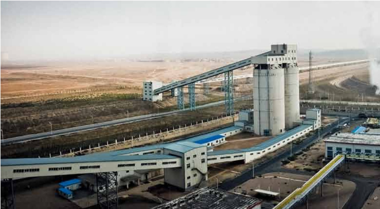
The olefins plant, at the heart of the Ningdong coal chemical center, represents an investment of US$2.8 billion – the largest-ever investment in Ningxia province.
