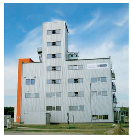
PLA pilot plant in Guben, Germany
