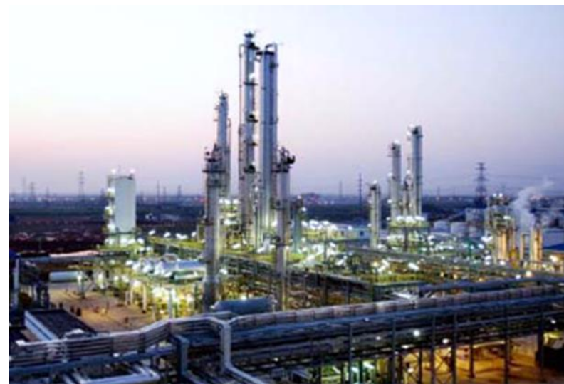
Najing Wison's 0.8 MMT merchant methanol to 0.3 MMT olefins plant
