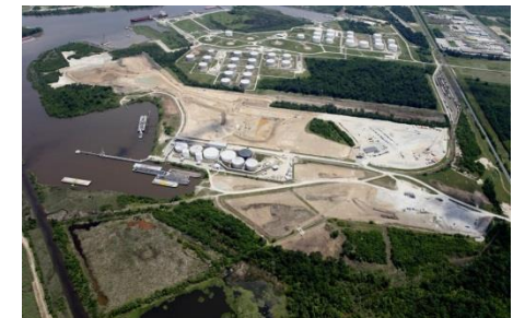
Natgasoline – aerial site view
