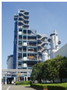
Used plastic gasification facility
