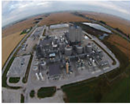
The DuPont biorefinery will produce biofuel from corn stover harvested within 30 miles of the plant.
