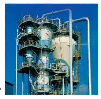
The core UNIPOL® PP process facility has the smallest footprint in the industry, about 60 meters by 65 meters. This includes the following operations:
