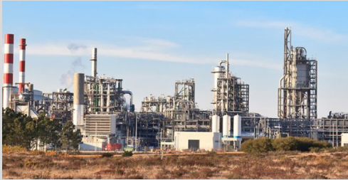
Artlant PTA, integrated with Artelia gas-based power plant
